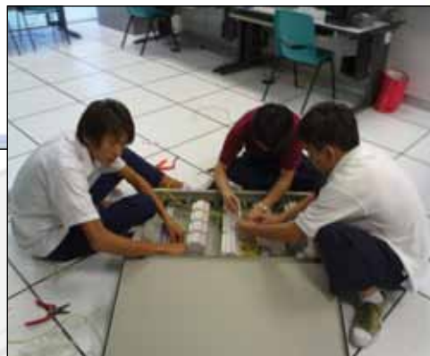
Students wire the KNX devices in the distribution box
