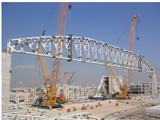
Fig. 1. A multi-crawler crane lift.
